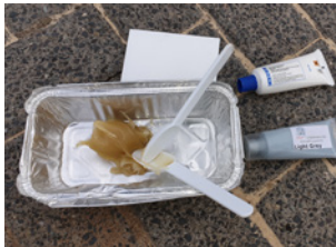
❾ Scoop out an appropriate amount of glue for the job in hand
