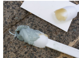
⓫ Using the plastic spoon fill in the clean holes. As the hardener is starting to take effect this needs to be completed within 10 mins
