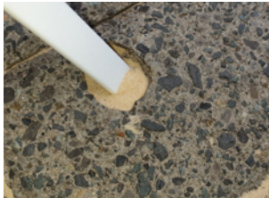
❺ Remove any debris or loose material from the hole
