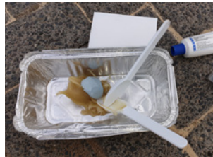
❿ Mix in the appropriate amount of colour pigment to match the subject area.
