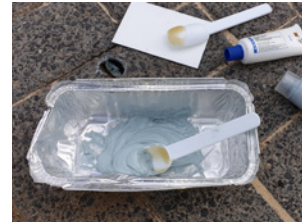
❼ Achieve the best colour match possible – ensuring the pigment is thoroughly mixed into the glue
