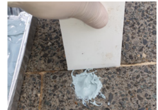
⓬ Fill the hole until the glue sits proud of the surface. Then use the plastic scraper to skim off to a smooth, flat surface
