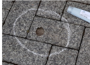
❷ Clearly mark the areas to be treated – once the hardener is added time is of the essence
